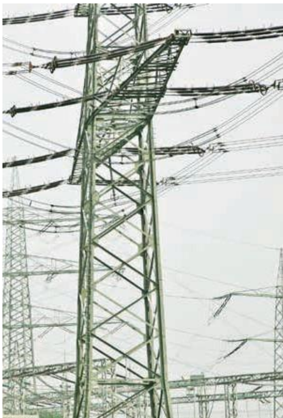
Pylons treated with a zinc dust paint based on Dynasytan® SIVO 140
