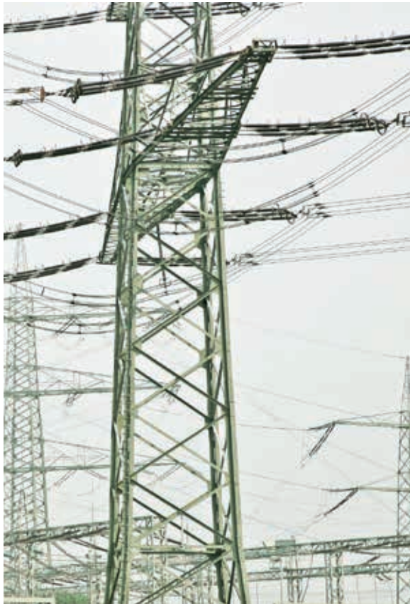
Pylons treated with a zinc dust paint based on Dynasylan® SIVO 140
